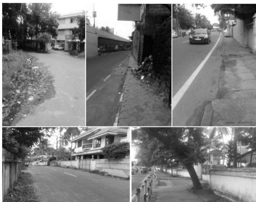
Figure 7. Condition of walk paths in Thiruvananthapuram City
